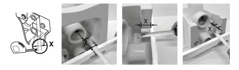
Measure the thickness of the ceramic 'X' from the support point of the WB9 B on the ceramic to the outermost point of the sanitary ware which will rest on the wall.
